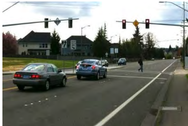
Enhanced Pedestrian Crossing with Pedestrian Signal
