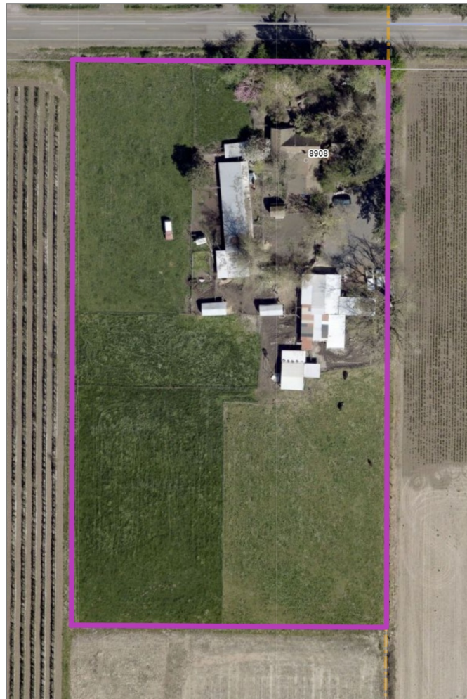
Close-up aerial image of the site (2021).
