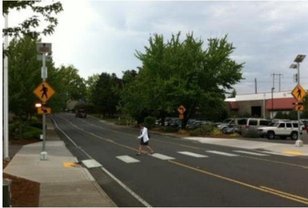
Enhanced Pedestrian Crossing with RRFBs
