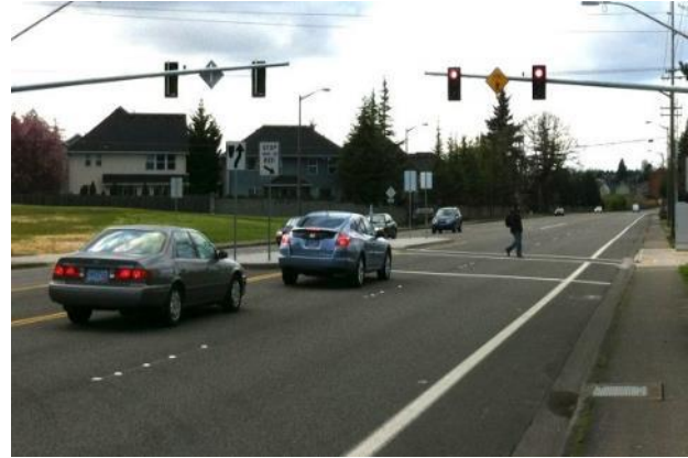
Enhanced Pedestrian Crossing with Pedestrian Signal
