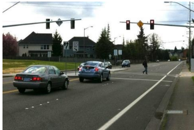
Enhanced Pedestrian Crossing with Pedestrian Signal
