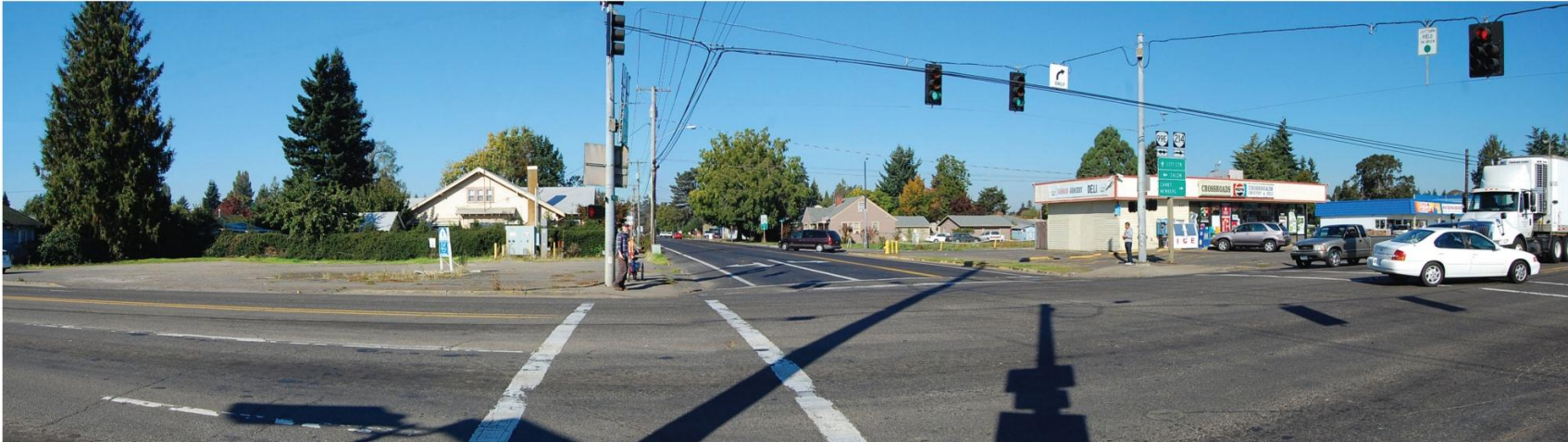
Young / Highway 99E Intersection (looking west): Before
