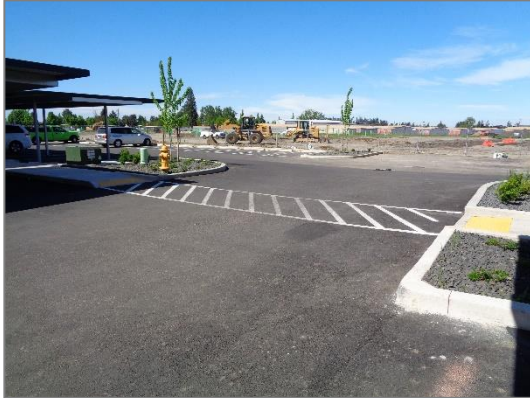
A-N: North walkway crossing
