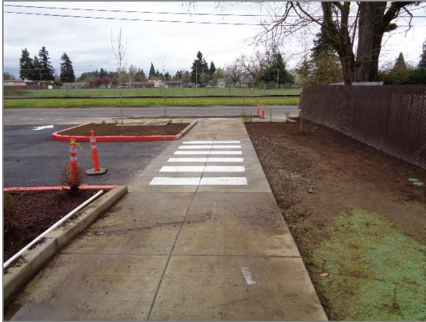
North cross access drive aisle as of March 28, 2024
