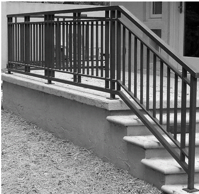
Exhibit 203B Example of railings having a bottom or near bottom horizontal member and a second horizontal member in addition to the top railing
