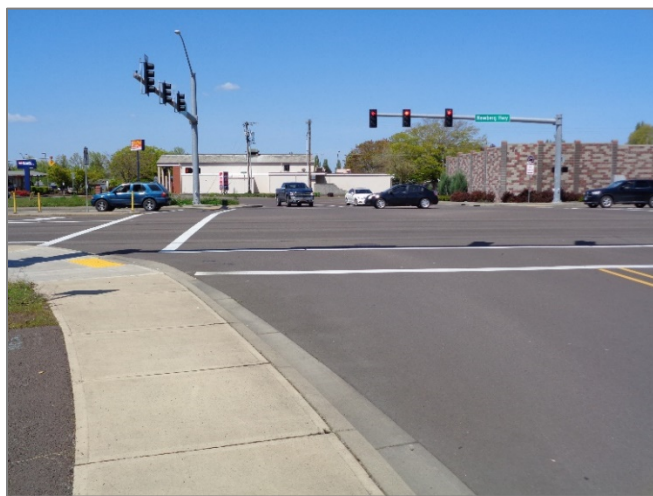
The turn lane from Oregon Way west onto Newberg Hwy. It is designed to accommodate large trucks.
