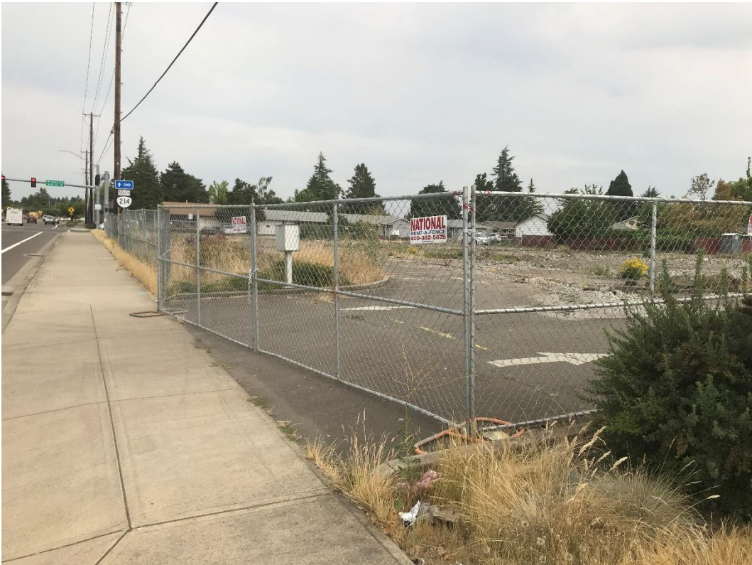
Figure 11. Newberg Highway right-in, right-out access facing east highlighting the straight and flat topography (to highlight potential pedestrian conflicts at the access).
