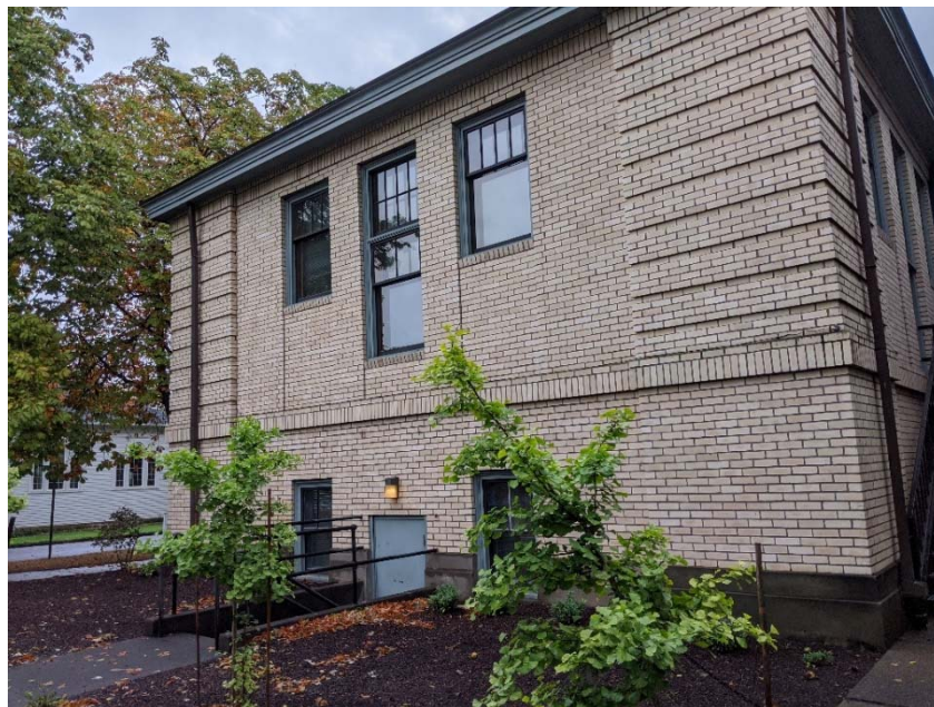
Figure 2: East Façade – Carnegie Library
