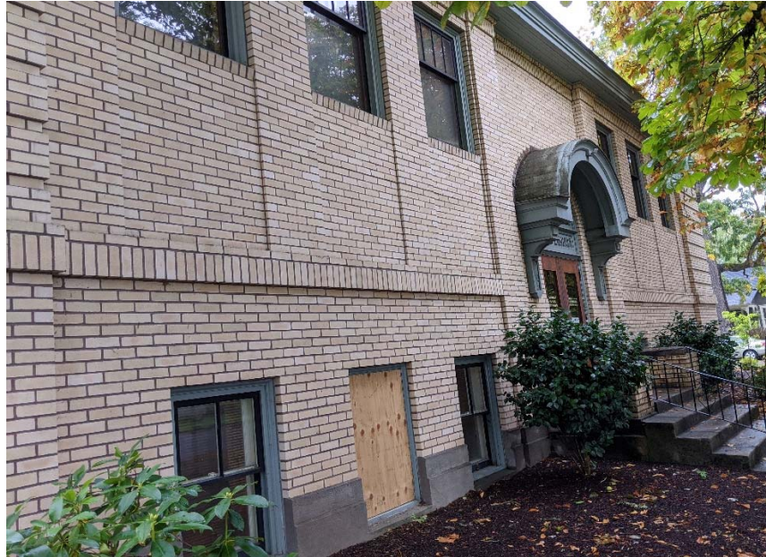
Figure 3: West Façade – Carnegie Library
