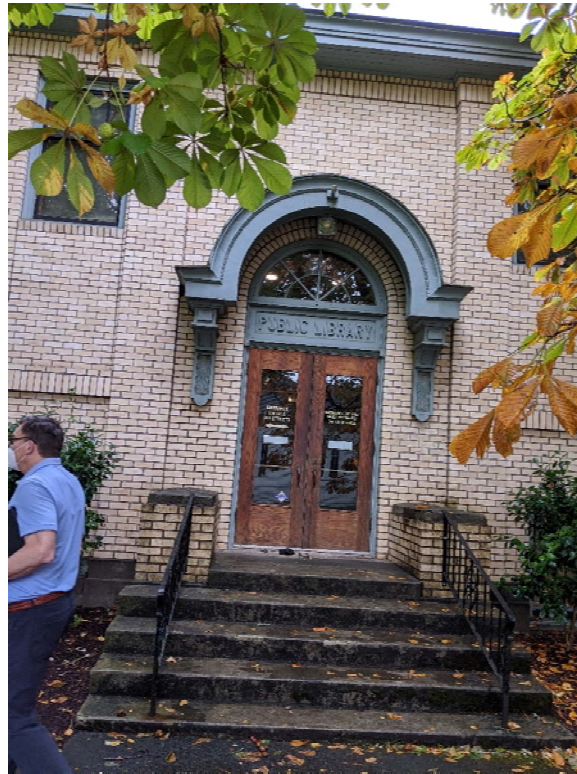
Figure 1: West Façade – Carnegie Library
