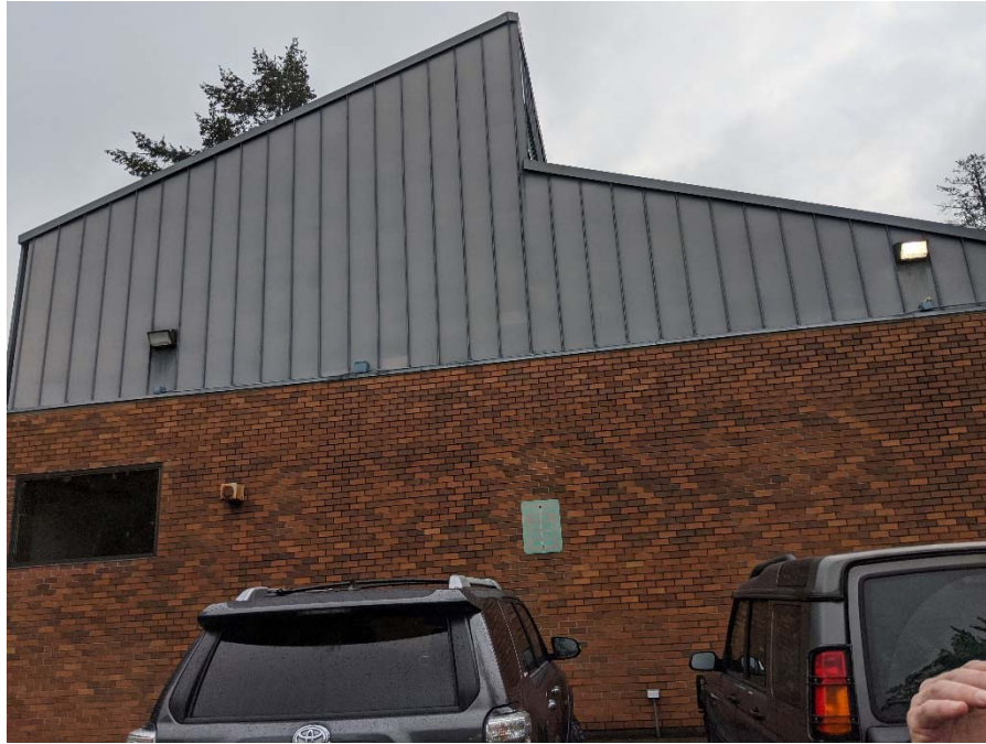
Figure 7: New Library South Facade
