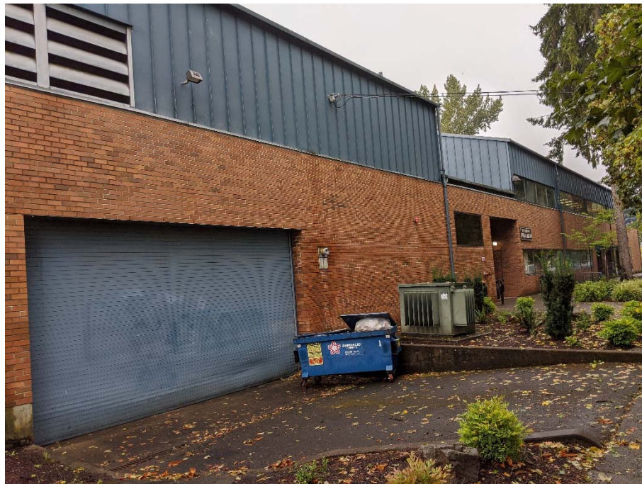
Figure 8: New Library – Westside at Loading Dock
