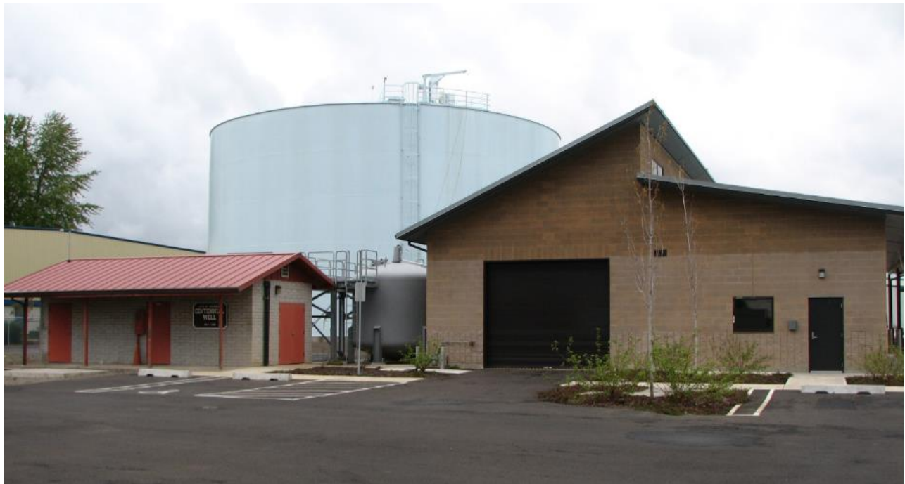
Centennial Well and National Way Water Treatment Plant
