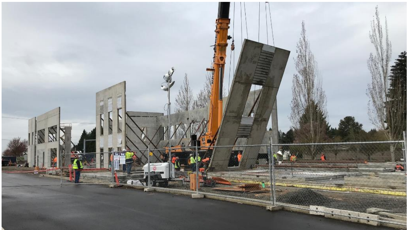
Construction of Salem Health Woodburn Clinic
