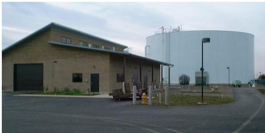
Water Treatment Plant at Country Club Road
