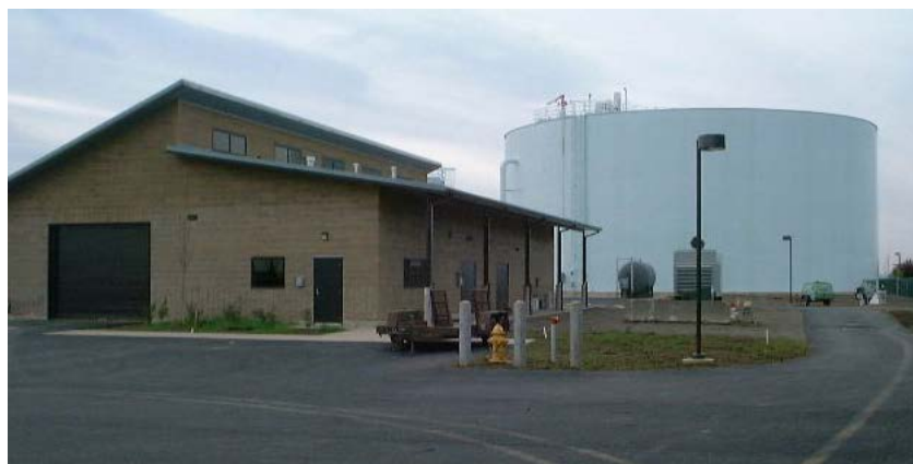
Water Treatment Plant at Country Club Road
