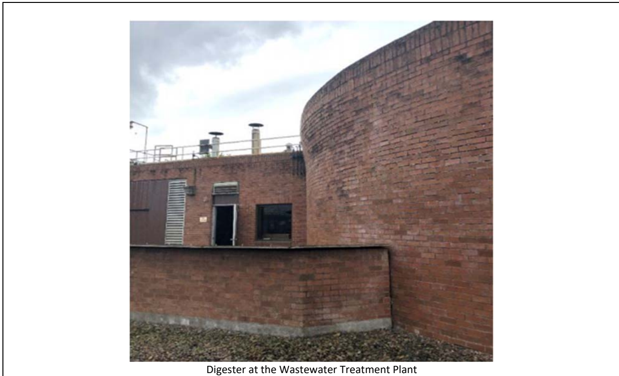
Digester at the Wastewater Treatment Plant
