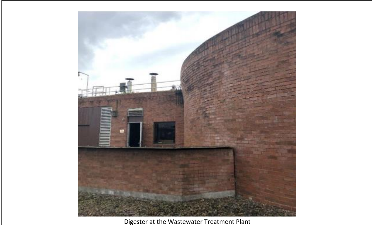
Digester at the Wastewater Treatment Plant
