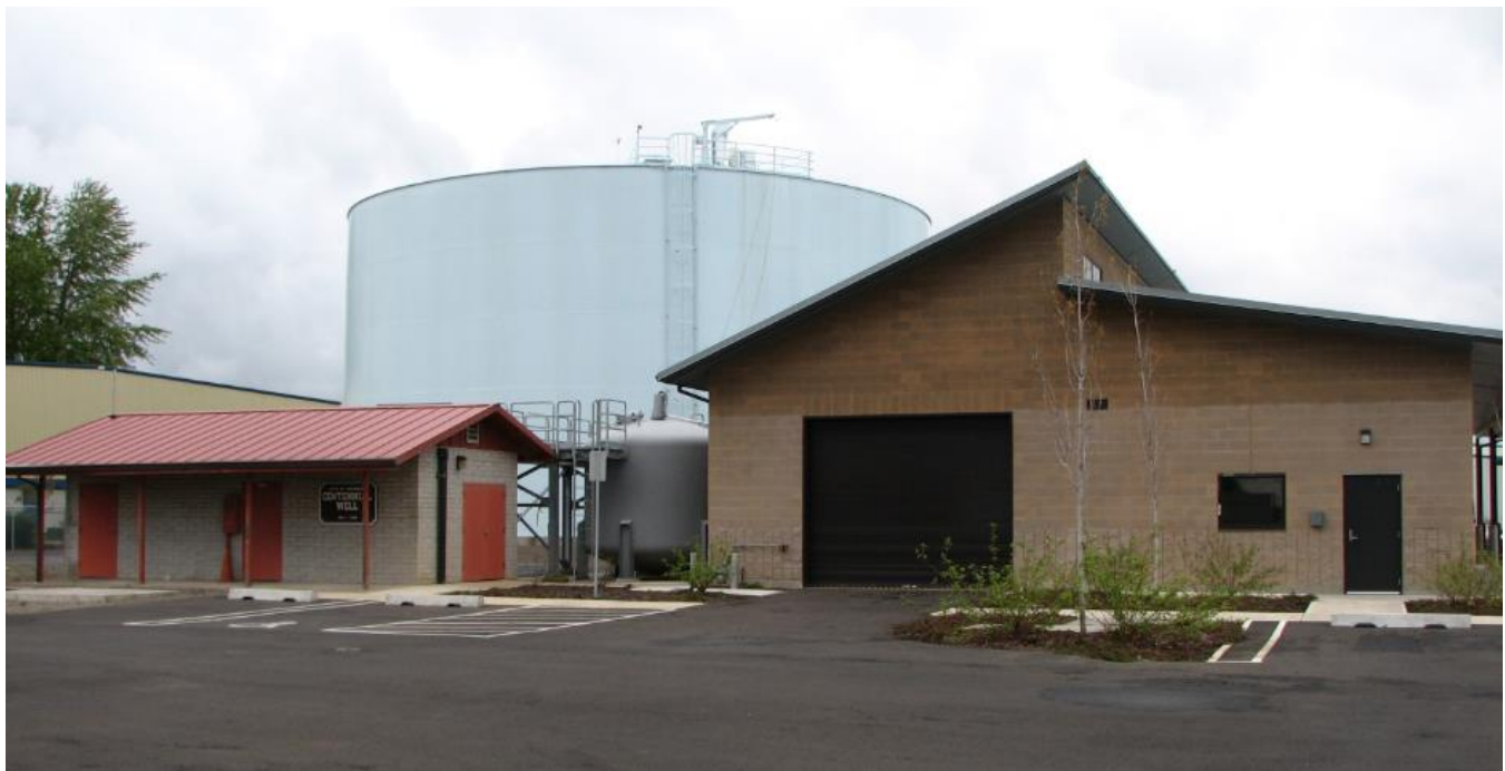
Centennial Well and National Way Water Treatment Plant
