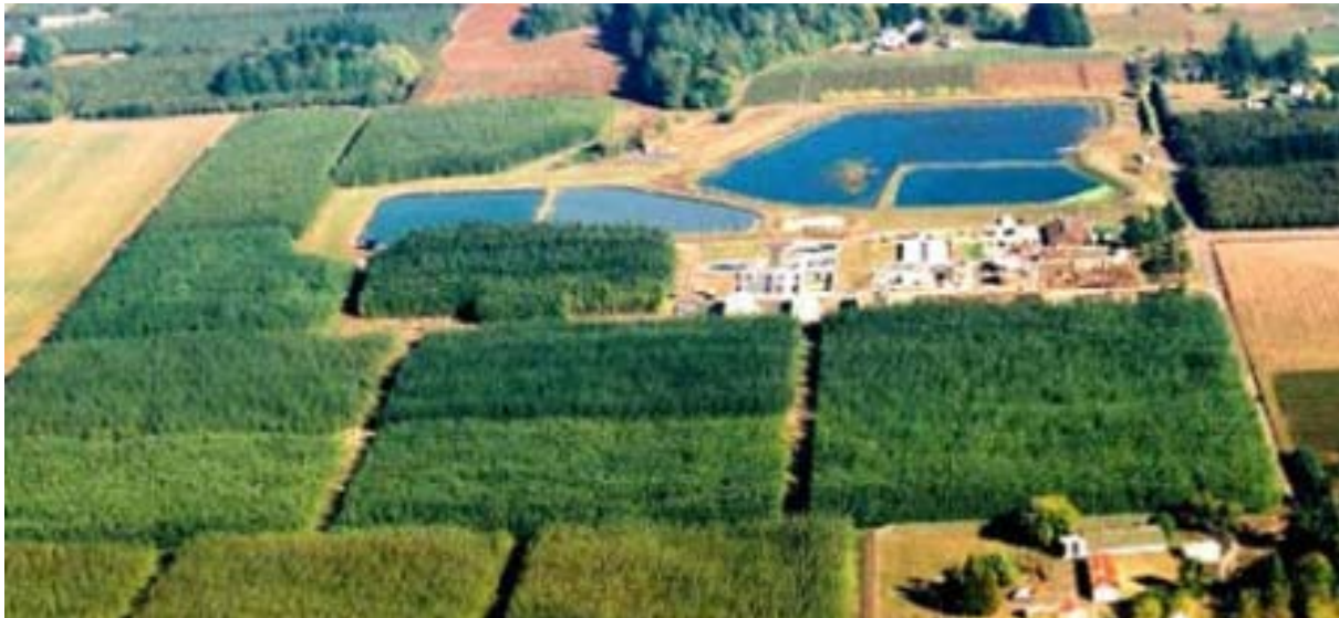
Aerial View of Wastewater Treatment Plant and Poplar Tree Plantation
