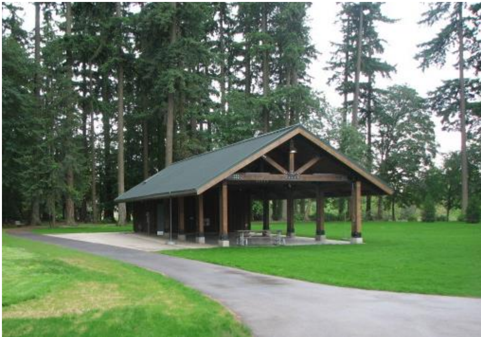
Legion Park Rehabilitation Project – New Pavilion - 2015
