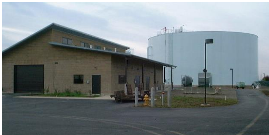
Water Treatment Plant at Country Club Road
