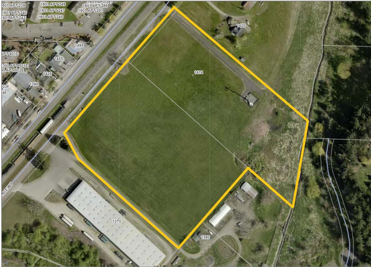
Aerial view of the site
