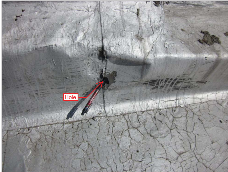
Sec. 1.03 – Roof A: View of hole in base flashing at north perimeter at the northeast section of the roof.
