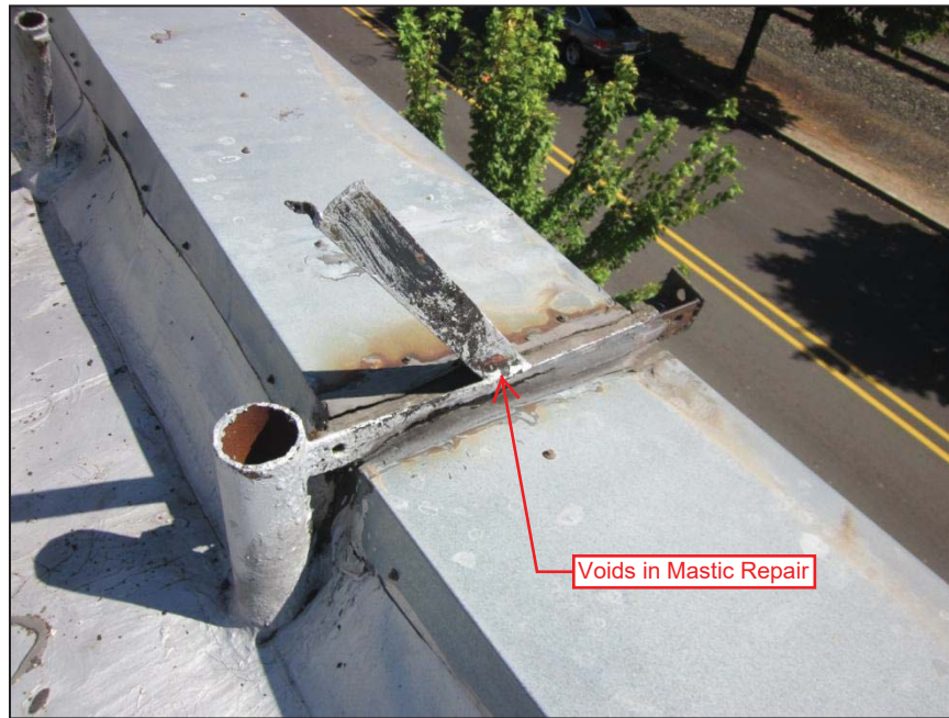
Sec. 1.05 – Roof A: View of typical void in previous mastic repair at metal coping joint at the east parapet.
