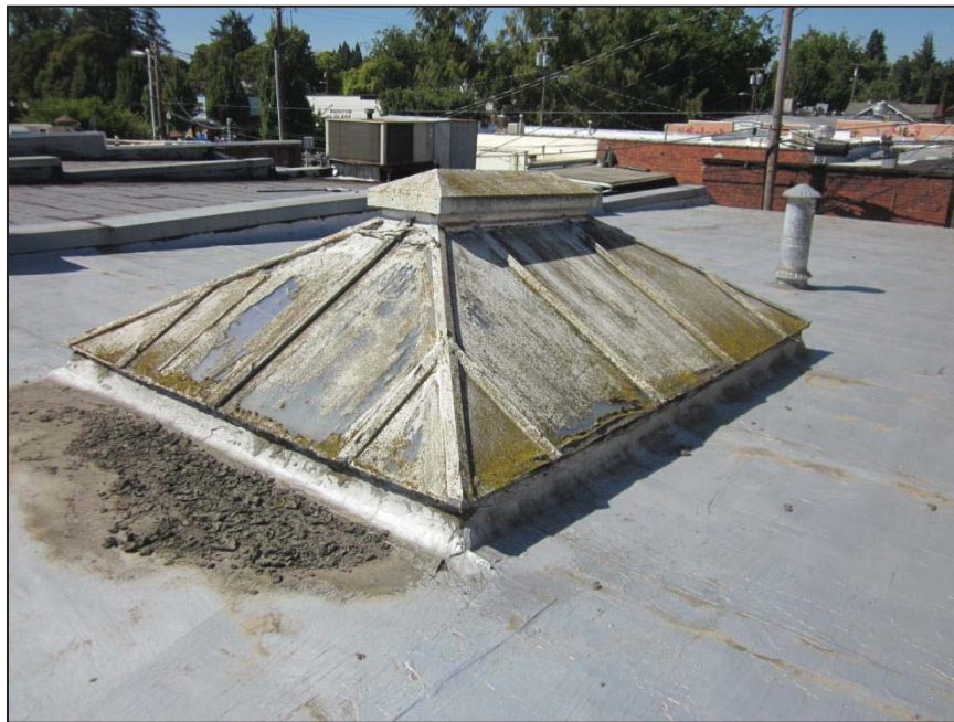
Sec. 1.10 – Roof B: View of skylight that has splits in membrane at base of skylight.
