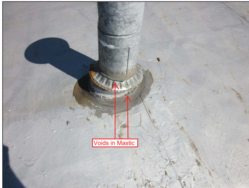
Sec. 1.11 – Roof B: View of voids in mastic repair at base of vent at the west section of the roof.
