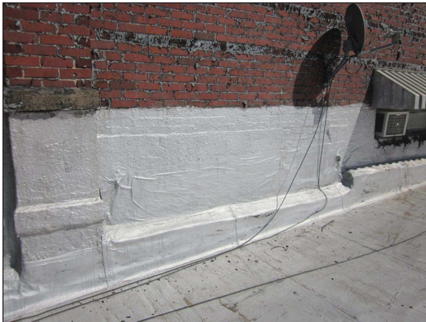
Sec. 1.08 – Roof A: View typical membrane and coating at the north perimeter.
