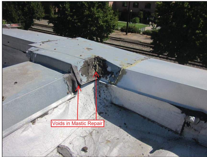
Sec. 1.09 – Roof B: View of voids in previous mastic repair to metal coping at the northeast corner of the roof.
