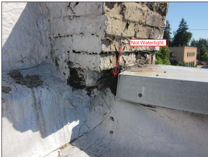
Sec. 1.04 – Roof A: View base flashing that is not watertight at the northeast corner of the roof.
